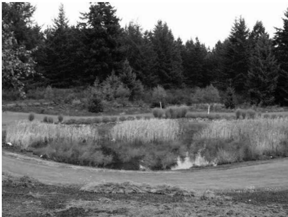
Infiltration Pond Along SR 510 in Thurston County.
