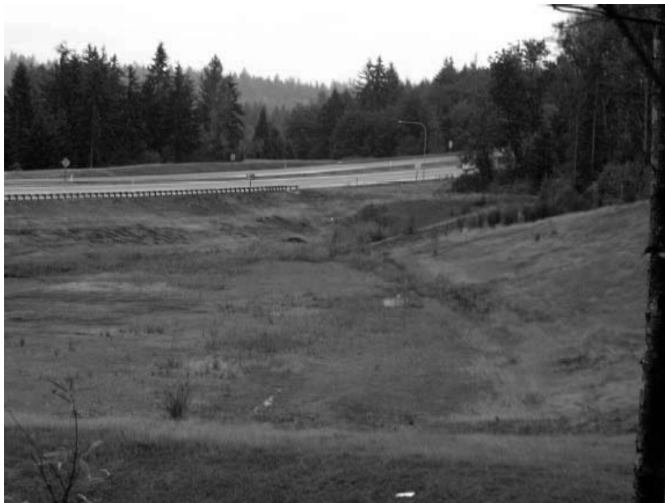
Detention Pond Along SR 18 in King County.
