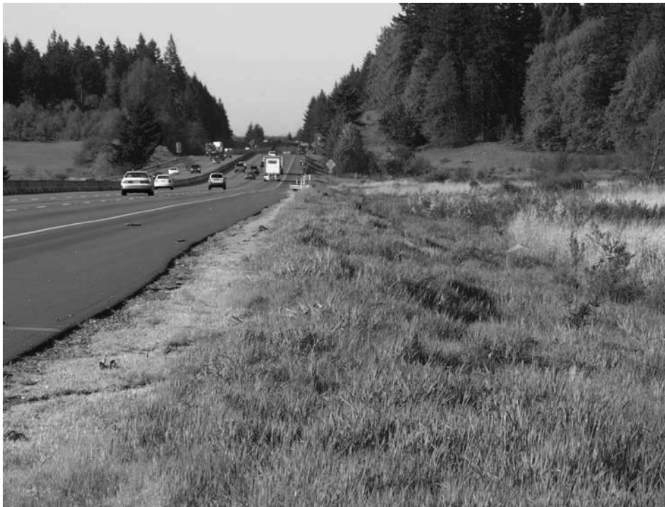
Engineered Dispersion Area Along I-5.
