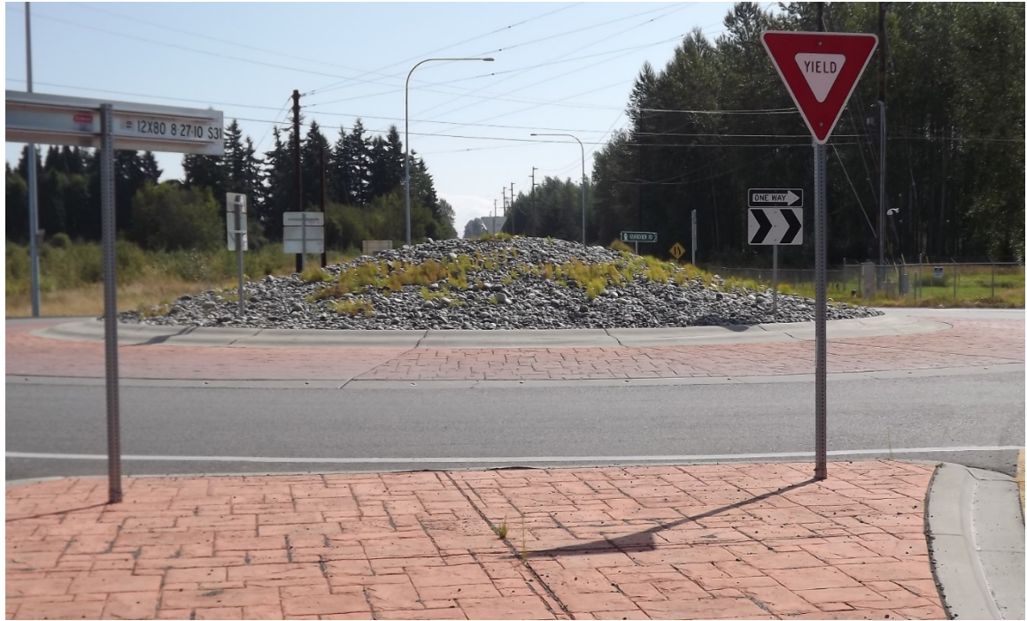
Roundabout with hardscape- reduces life cycle/maintenance costs.
