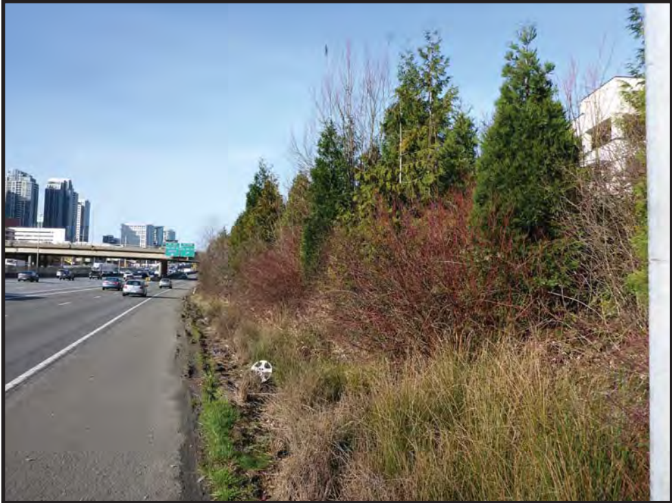
Figure 22. Zone 81 A1, view to the northwest. Note runoff along edge of pavement and dense vegetation.
