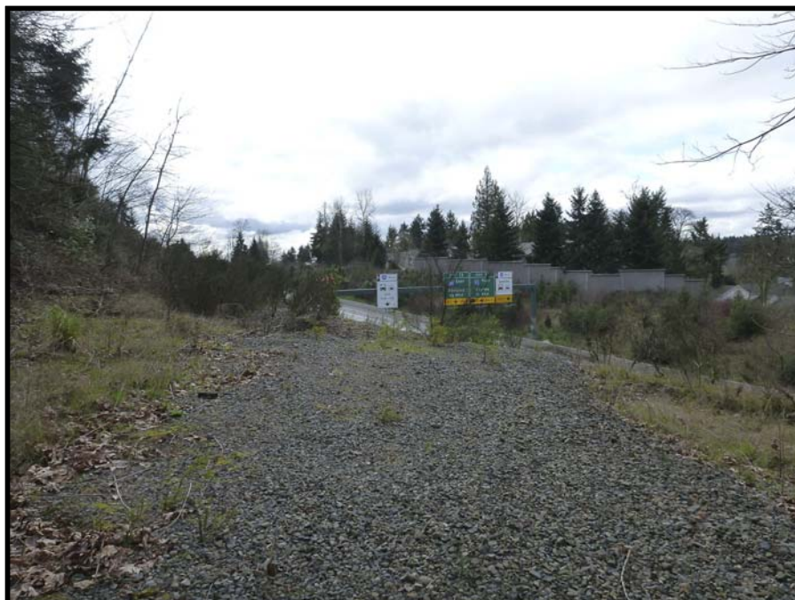
Figure 3. Photograph showing the railroad bed and the location of the former Wilburton tunnel, view to the southwest.
