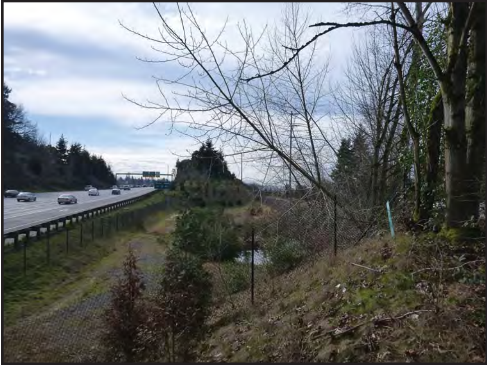
Figure 5. Photograph showing one of the water retention ponds. Note how I-405 is cut into the side of the hill, view to the south.
