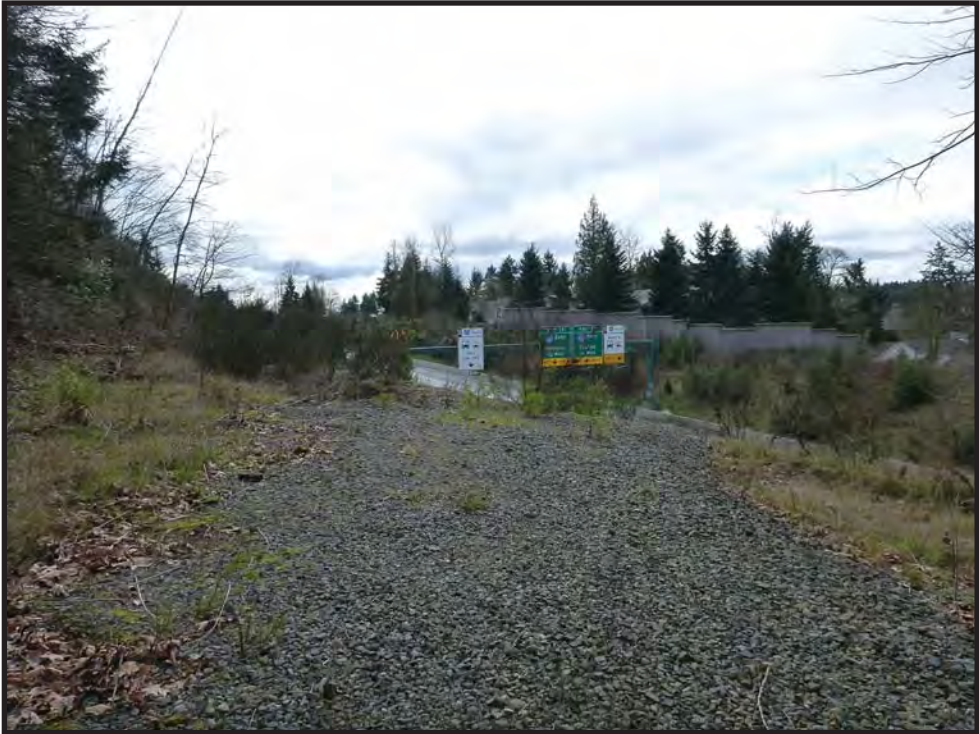
Figure 12. Photograph showing a segment of the abandoned railroad bed overlooking the former location of the Wilburton Tunnel, view to the southwest.
