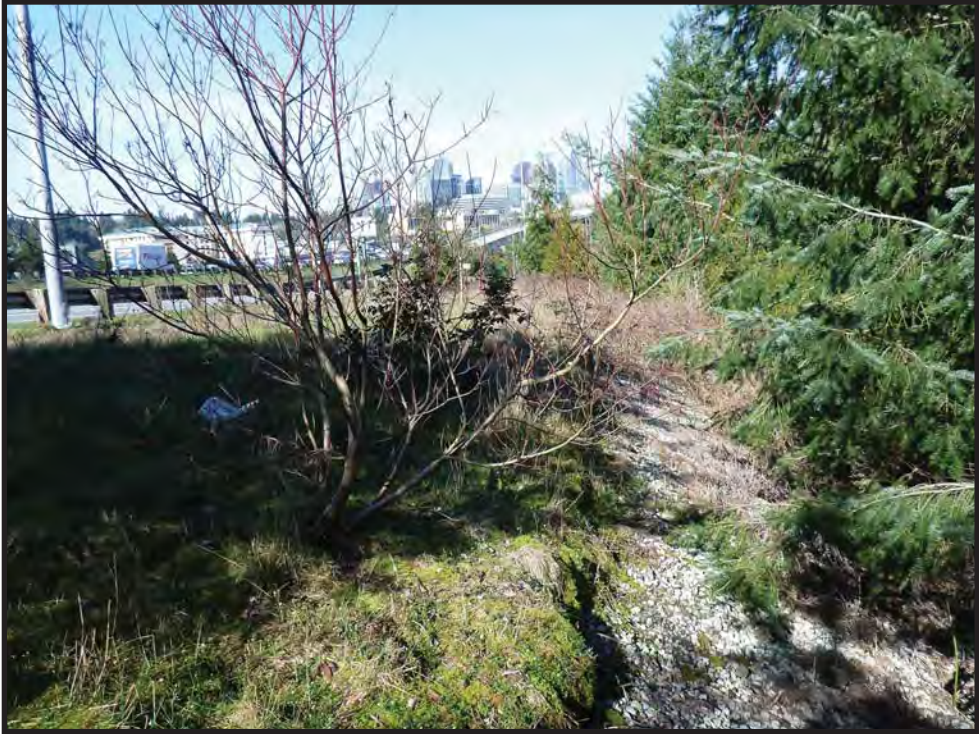
Figure 11. Zone 69 A2, view to the northwest. Note gravel layer on slope under grass mat.
