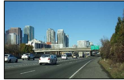
Existing Main Street Overpass
