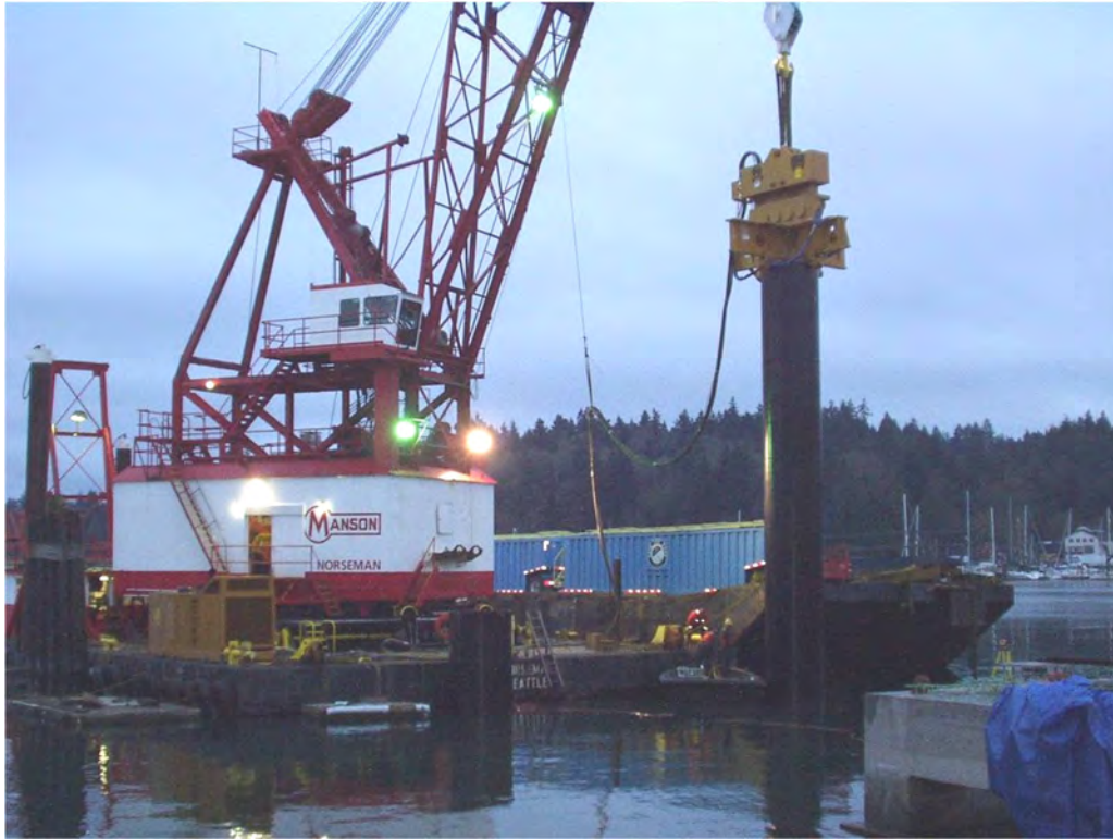
Figure 2-9 Vibratory Installation of Drilled Shaft Casing
