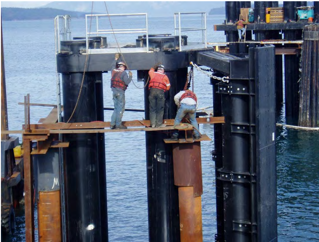
Figure 2-51 Work Platform Supported by Temporary Steel Piles
