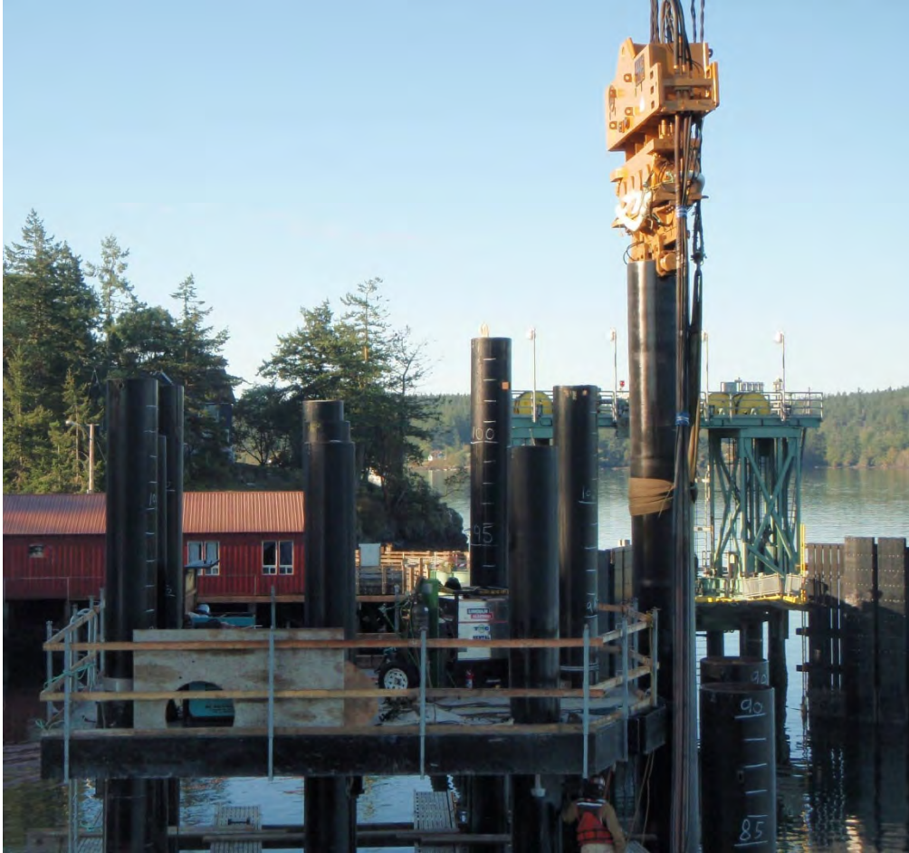
Figure 2-5 Vibratory Hammer Installing a Steel Pile
