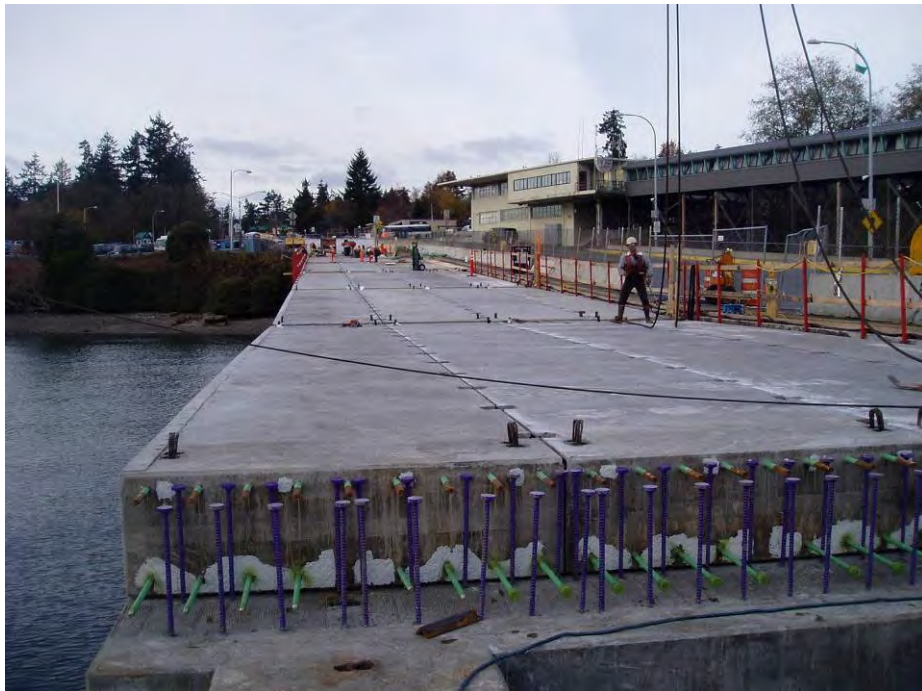
Figure 2-46 Pre-cast Concrete Deck Panels
