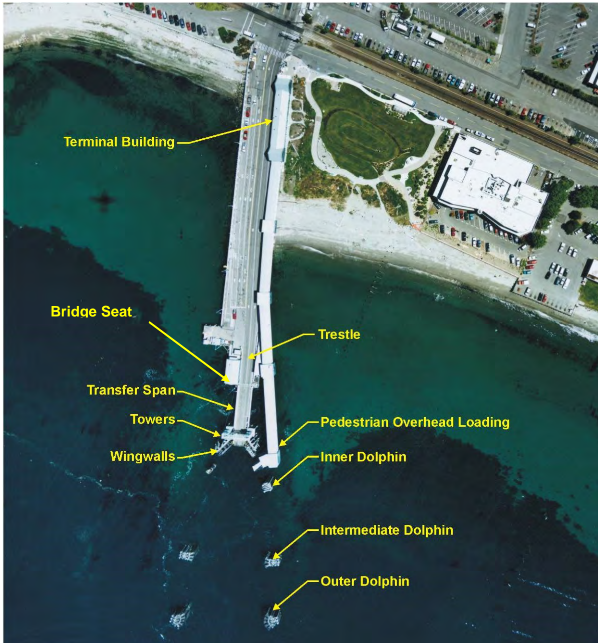
Figure 2-23 Typical Ferry Terminal, Aerial View
