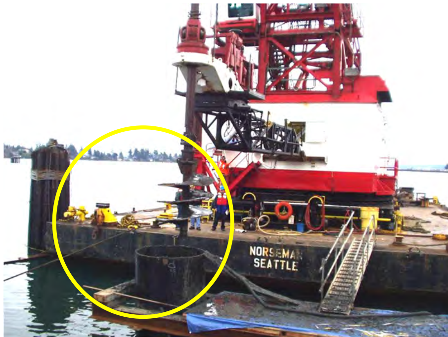
Figure 2-10 Auger Excavation of Drilled Shaft
