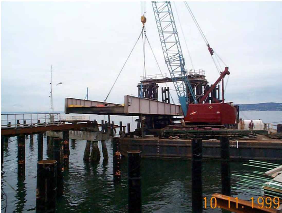
Figure 2-39 Removal of a Transfer Span
