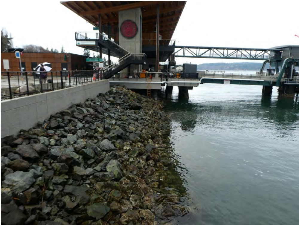
Figure MU-10 Shoreline near Terminal Building looking SW.
