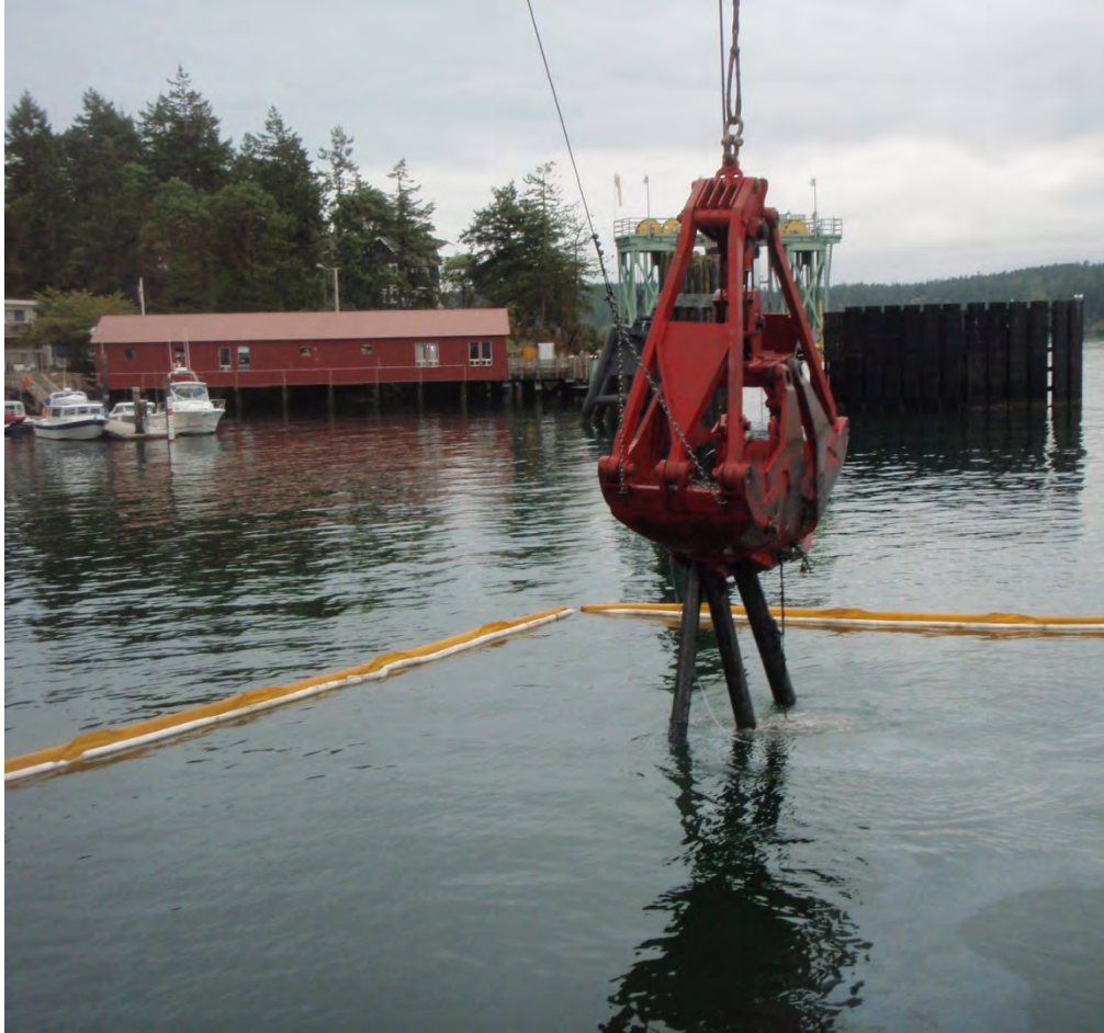
Figure 2-3 Removal of a Broken Pile with a Clamshell Bucket
