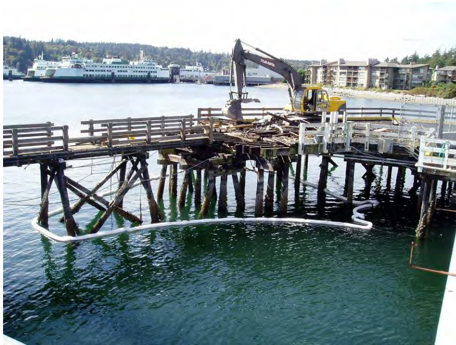
Figure 2-43 Removal of Timber Decking
