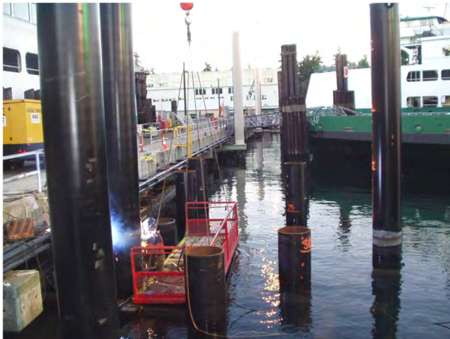
Figure 2-21 Bent Steel Pile in Need of Repair
