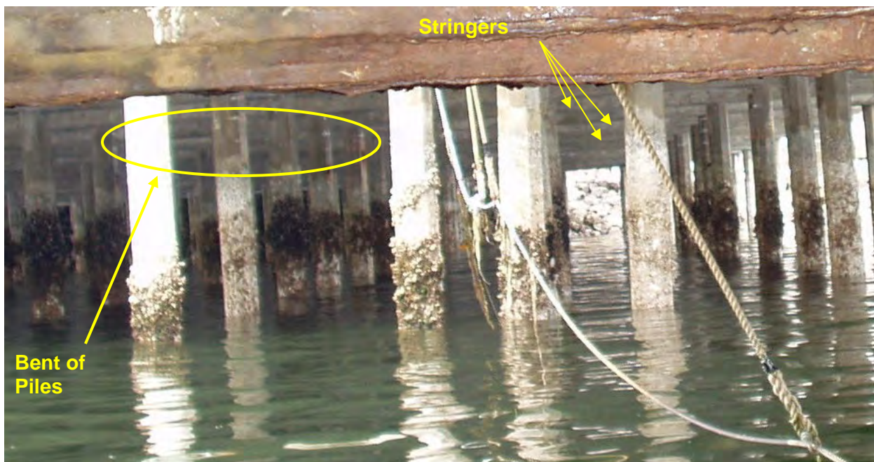
Figure 2-42 Under a Timber and Concrete Trestle
