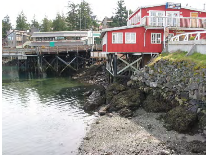
Figure FH-3 Shoreline Area on the Northwest Side of the Friday Harbor Ferry Terminal
