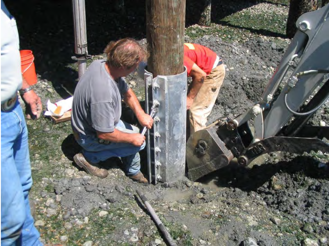
Figure 2-15 Pile Stubbing: Steel Collar Method
