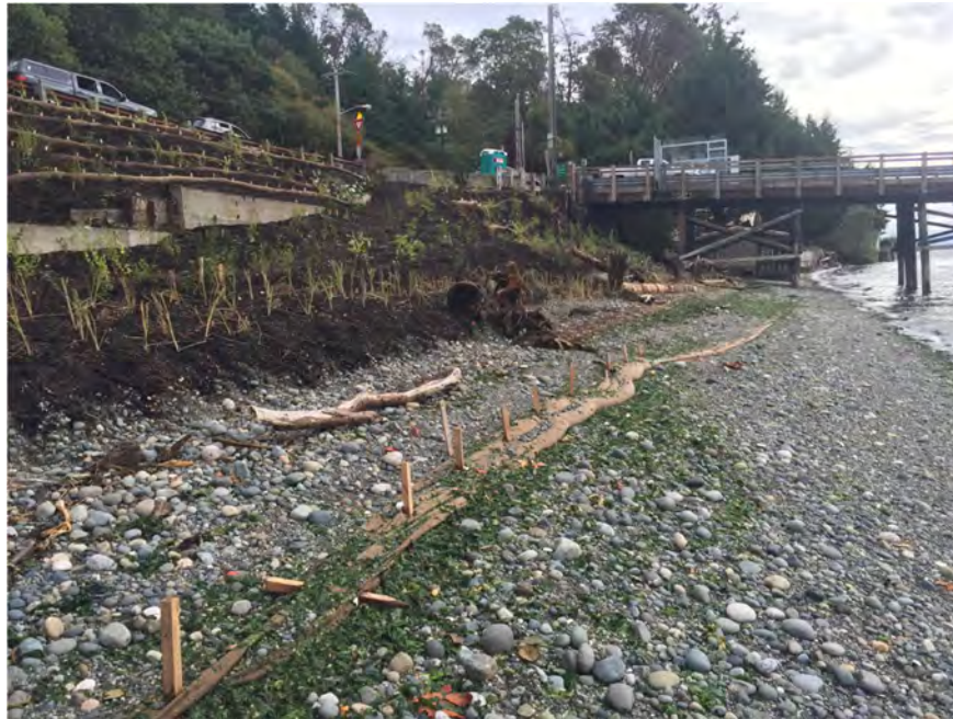
Figure TA-5 Shoreline West toward the trestle post soft-shore project
