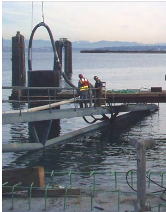
Figure 2-12 Vacuuming of Slurry from Drilled Shaft
