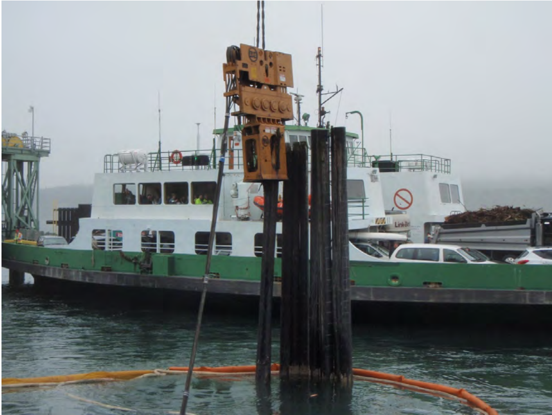
Figure 2-1 Vibratory Hammer Removing a Timber Pile
