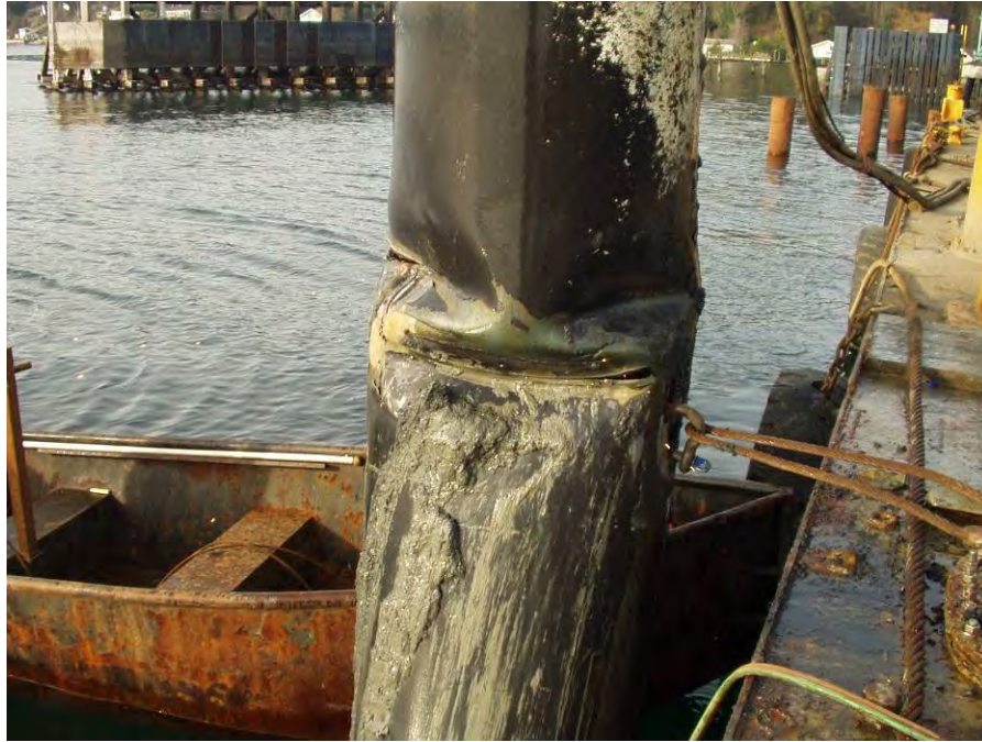
Figure 2-21 Bent Steel Pile in Need of Repair
