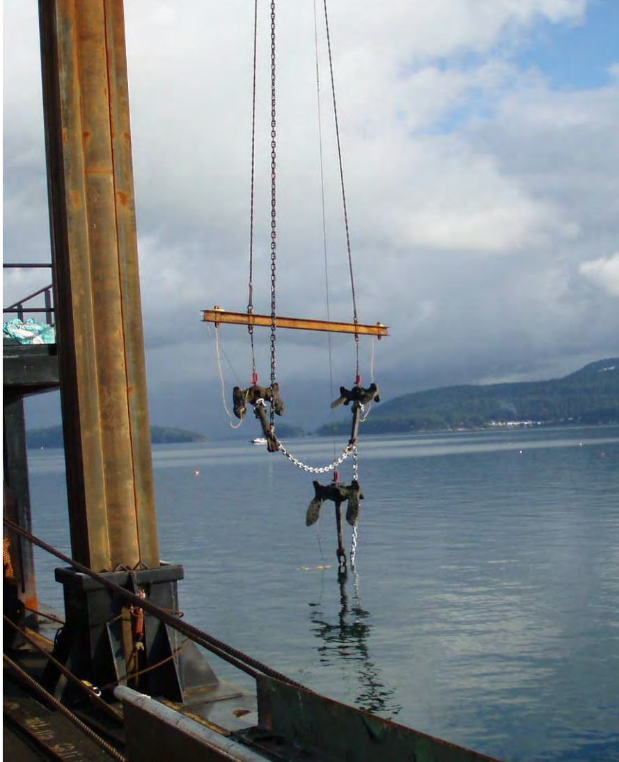
Figure 2-29 Installation of Floating Dolphin Anchors
