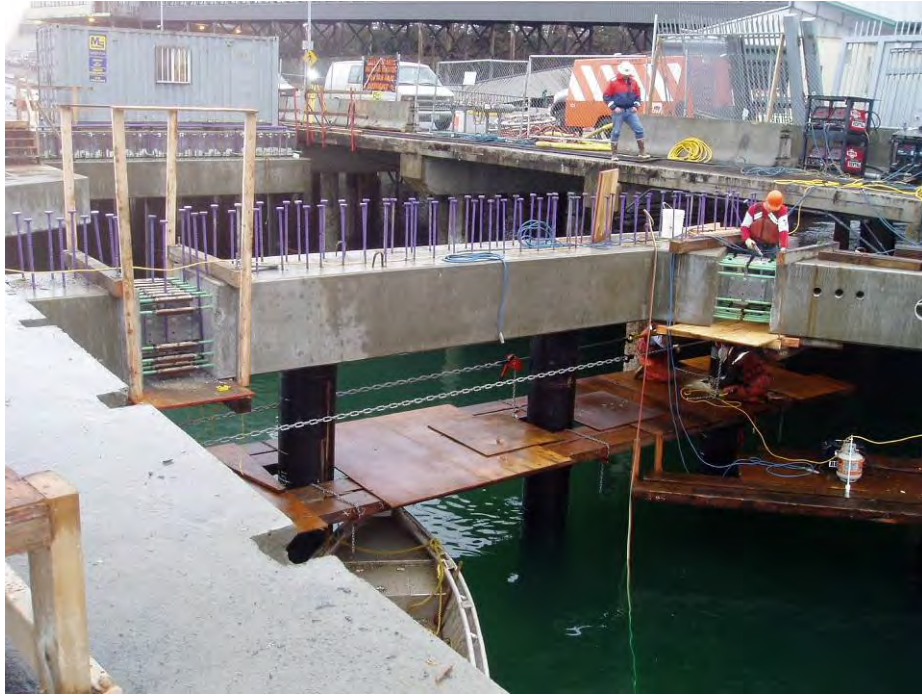
Figure 2-44 Concrete Pile Cap
