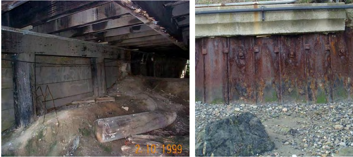
Figure 2-49 Timber and Steel Bulkheads
