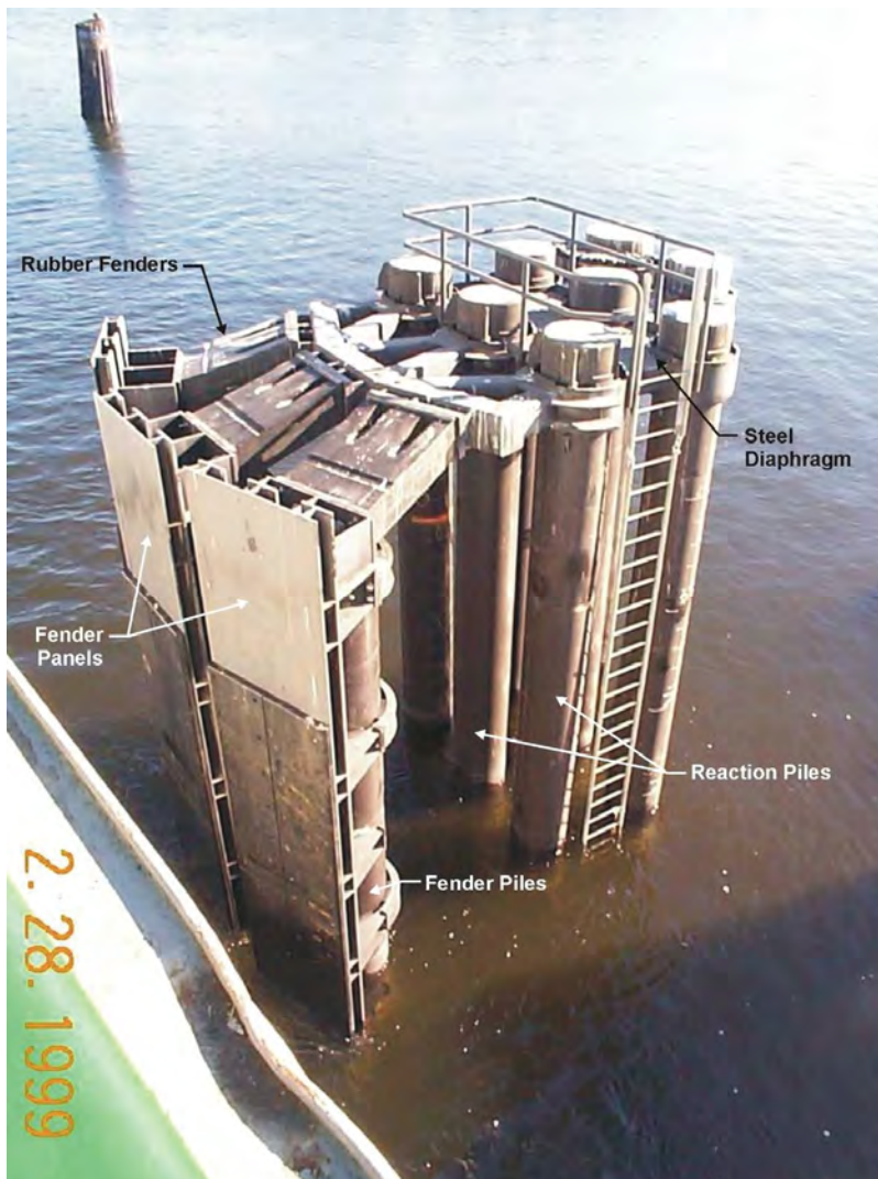
Figure 2-31 Typical Steel Dolphin
