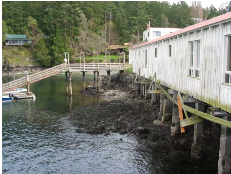
Figure SH-4 Shoreline Area East of the Shaw Island Ferry Terminal
