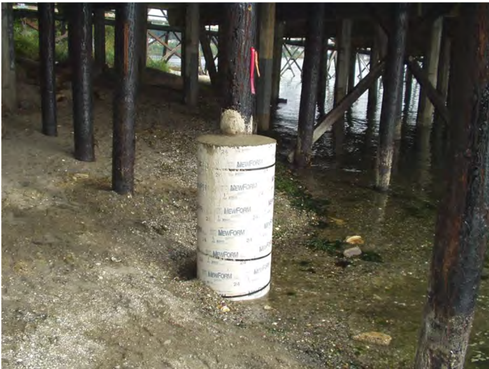
Figure 2-19 Completed Pile Encapsulation
