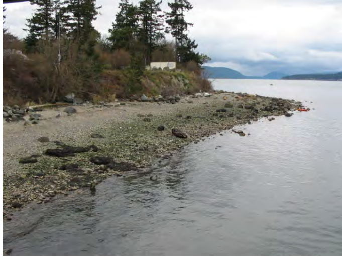
Figure AN-3 Shoreline Area to the West of the Anacortes Ferry Terminal
