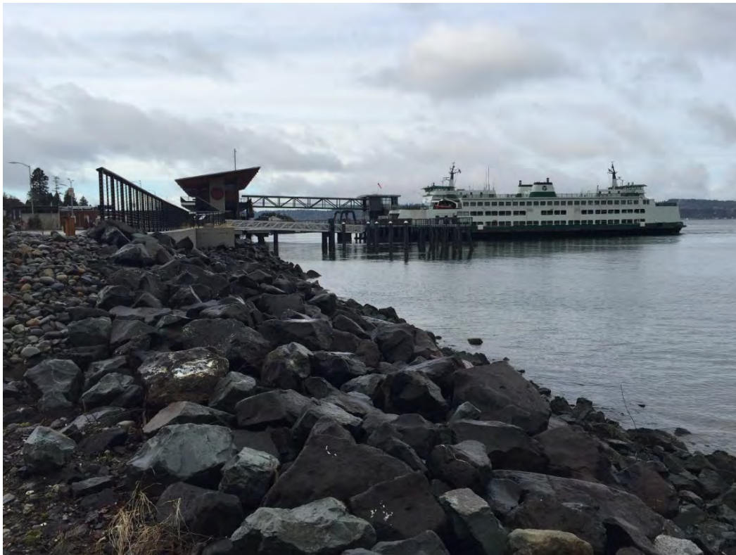
Figure MU-8 Shoreline from the NE boundary of the terminal looking SW
