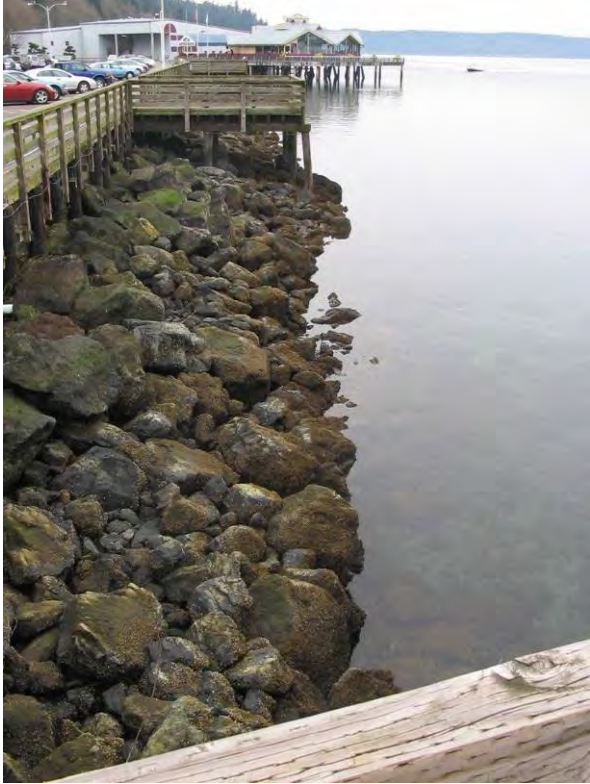
Figure PD-3 Shoreline South of the Point Defiance Ferry Terminal
