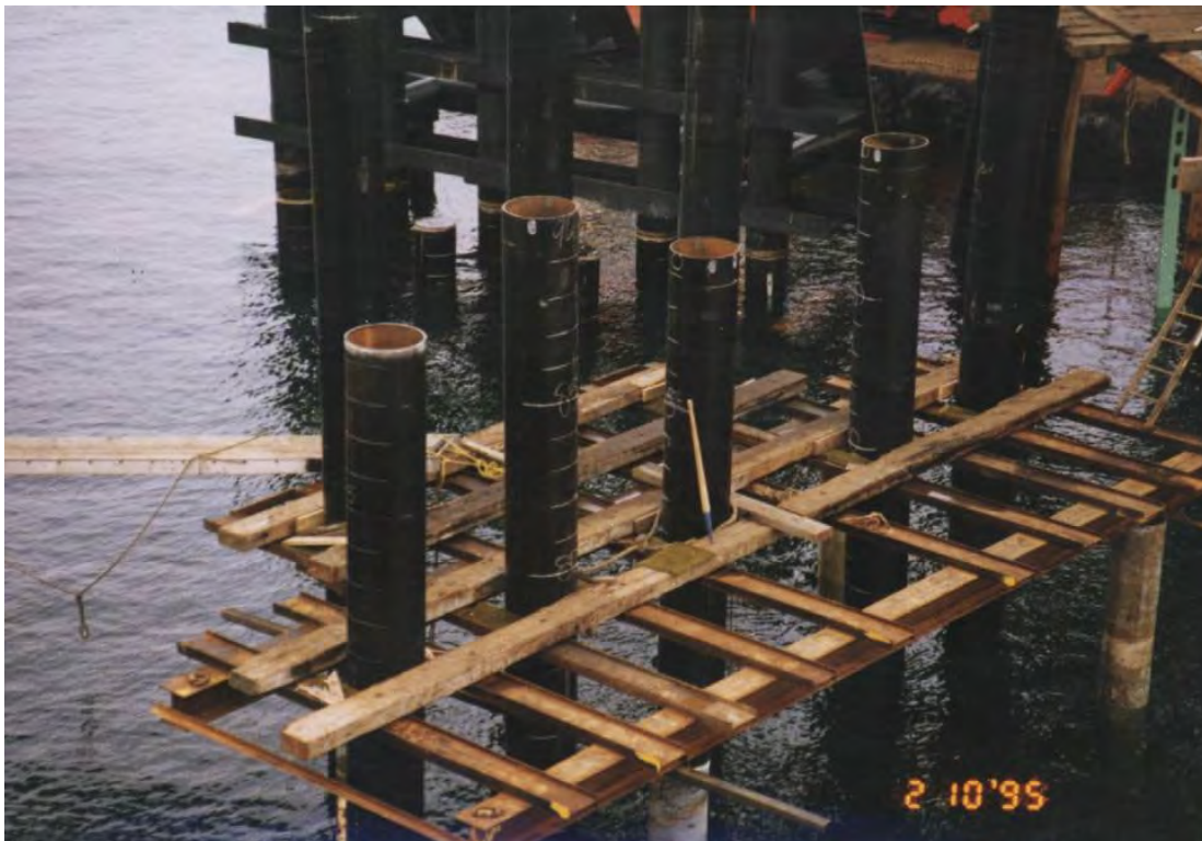
Figure 2-36 Template Used During Steel Wingwall Installation
