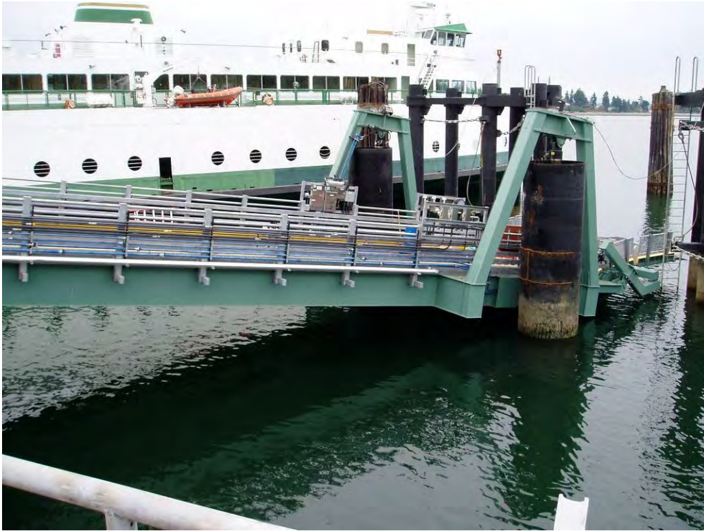
Figure 2-38 Compression Cylinder Tower System
