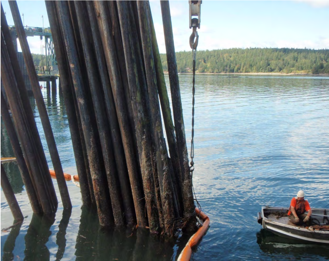
Figure 2-2 Direct Pull of Timber Piles
