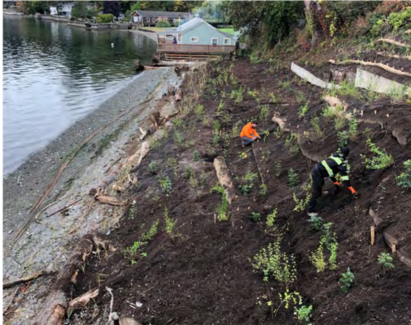
Figure TA-4 Shoreline West of the trestle post soft-shore project
