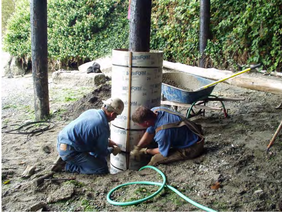
Figure 2-18 Installing the Form
