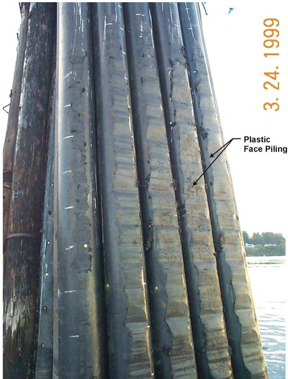
Figure 2-27 Plastic Face Piling on a Fixed Timber Dolphin
