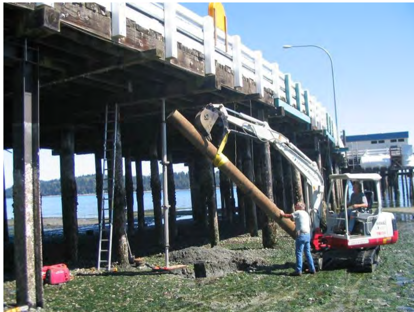
Figure 2-14 Pile Stubbing: Setting New Pile Section in Place
