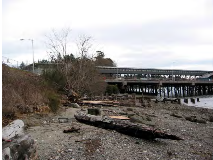
Figure BA-3 Beach Area on South Side of Bainbridge Island Ferry Terminal
