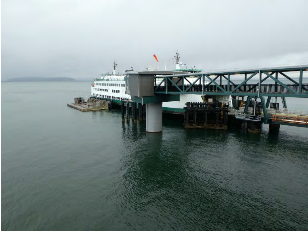
Figure MU-7 Hydraulic Transfer Span, Wingwall, Overhead Loading, Fixed Dolphin, Floating Dolphin
