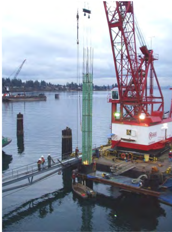
Figure 2-11 Rebar Reinforcement of Drilled Shaft
