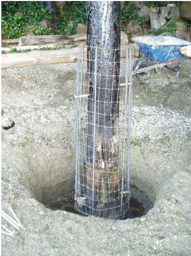
Figure 2-17 Pile Prepared for Encapsulation
