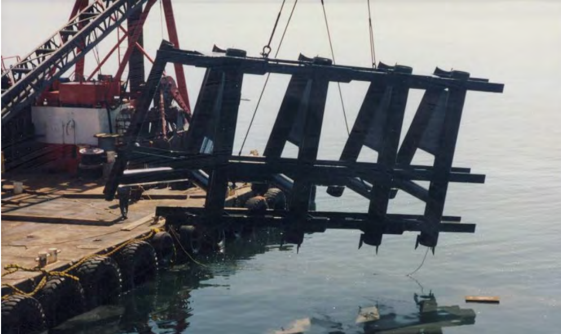
Figure 2-37 Crane Installing Steel Wingwall Frame
