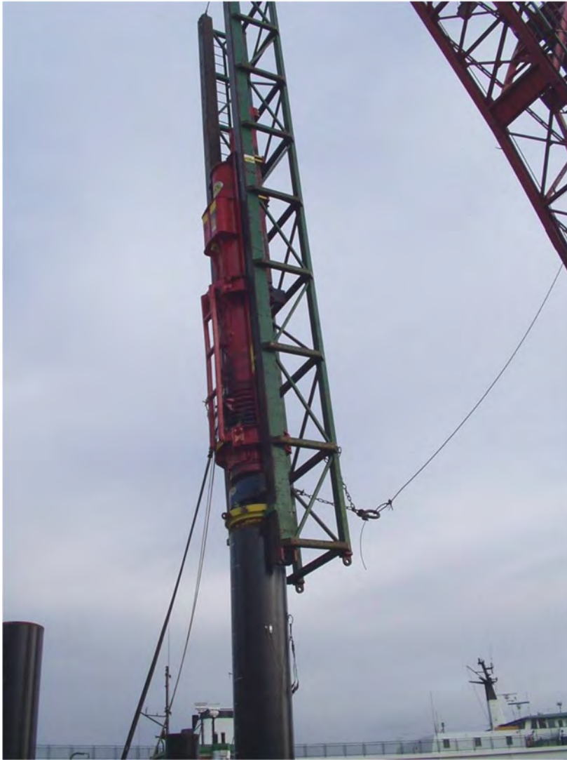
Figure 2-4 Impact Hammer Driving a Steel Pile
