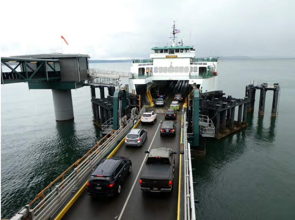
Figure MU-6 Hydraulic Transfer Span, Wingwalls, Fixed Dolphins, Overhead Loading
