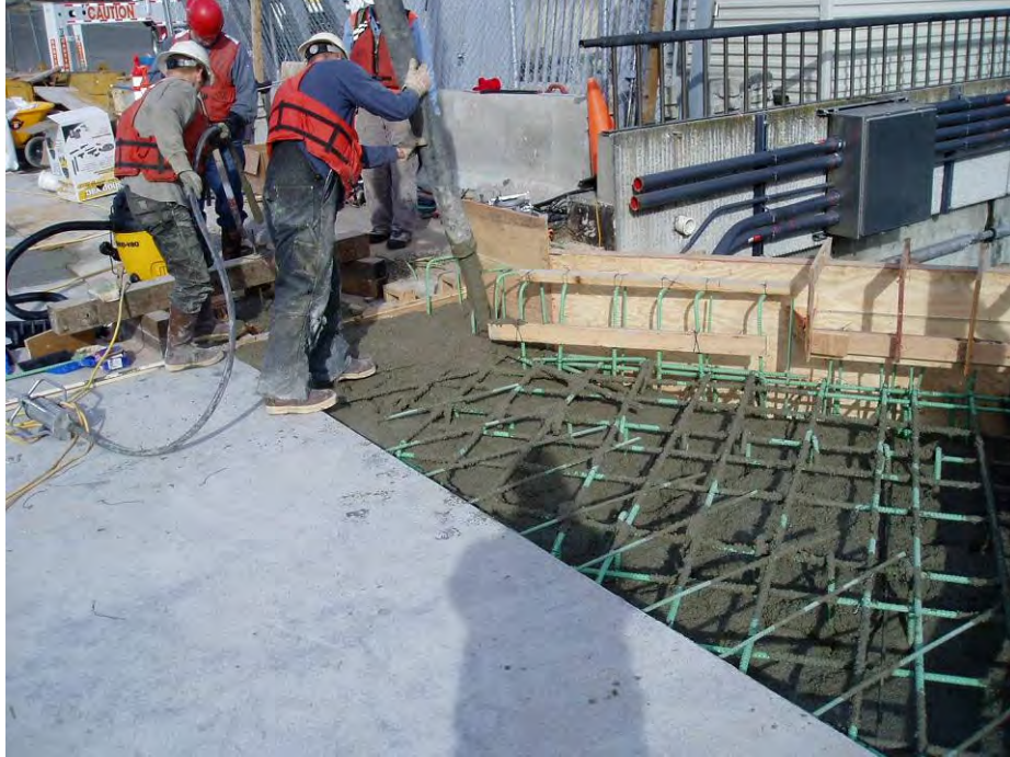
Figure 2-45 Pouring Concrete for Cast-in-place Deck Panels
