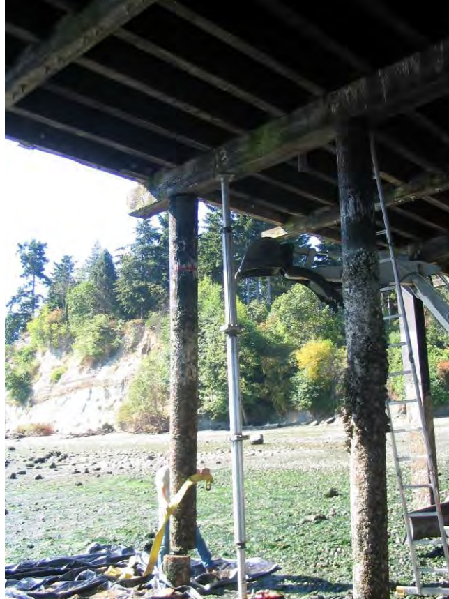
Figure 2-13 Pile Stubbing: Removing a Damaged Section of Pile
