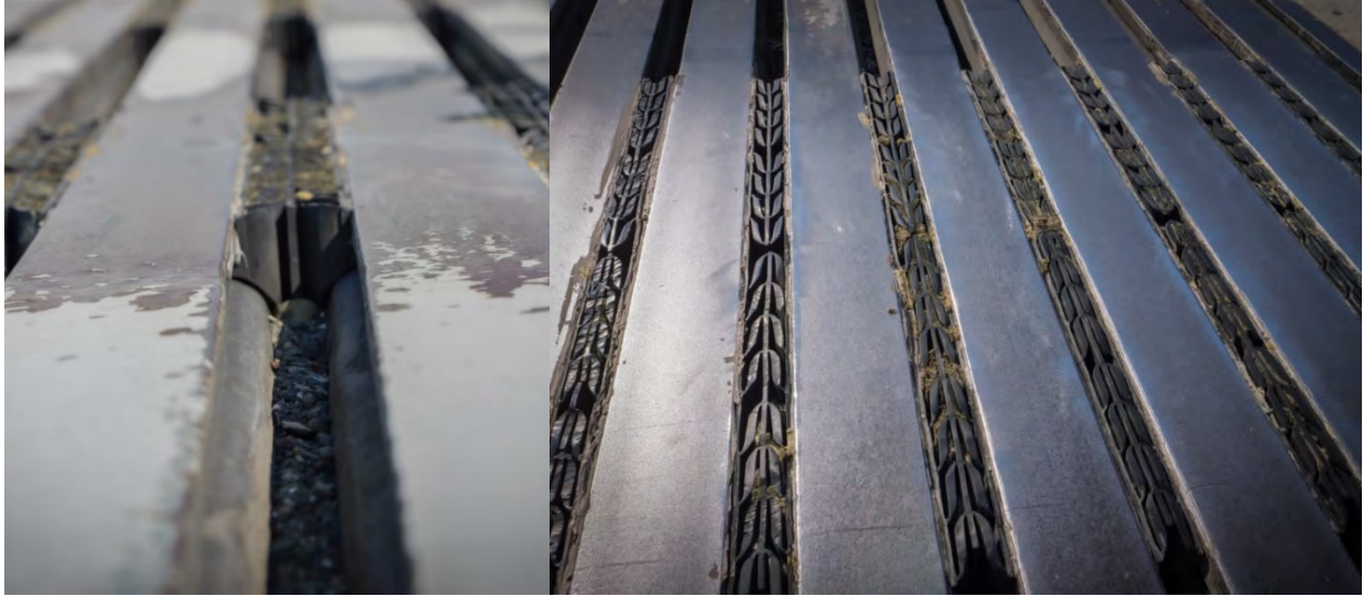
Figure 4-11. Over one month of installation, gravel and debris started to fill up the unsupported portion of the joint (left), while we observed no debris in the chevrons themselves. While the chevrons remained in good condition, some foam had been pulled from the supports after one month of wear (right).
